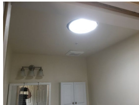
Sola-tube in bathroom interior
