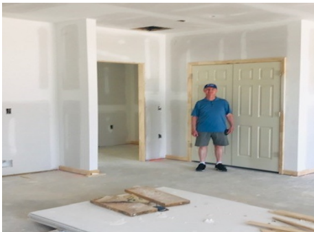
Drywall construction: main living area.
