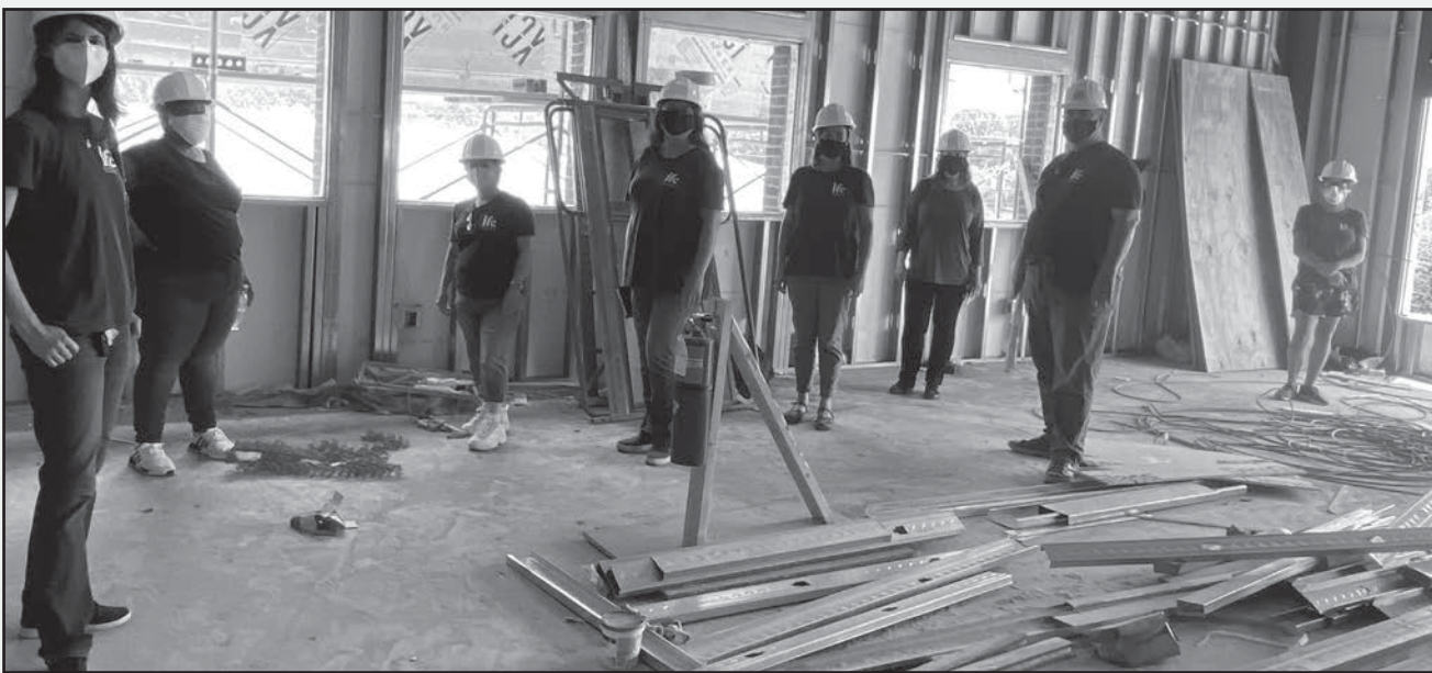
IFC staff team members take a tour of the building under construction.
