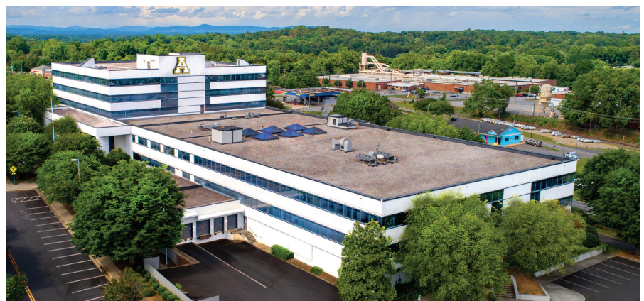
Concept art provides an aerial view of the former Corning Optical Communications building in Hickory. The six-story, 225,800-square-foot facility is the largest in App State's building portfolio.
