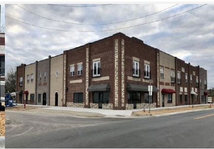
Fair Bluff Uptown Completed June 2024
