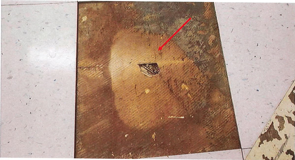
Photograph 1 - Homogeneous Area A-06—Typical Asbestos-Containing 9" x 9" Floor Tile (Green & Brown) with Black Mastic Located Under Carpet or Non-ACM Floor Tile in Waiting Room, Exam Rooms, etc. See Drawing Attached in Appendices for Exact Locations. (2,600 SF)
