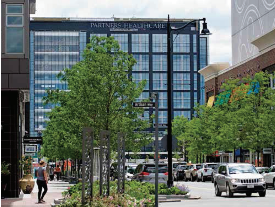
← Partners Healthcare's new Assembly Row facility in Boston incorporates energy-efficient technologies, hosts a 1.25 MW solar array on the rooftop of its parking garage and is a LEED Gold Version Four candidate.
