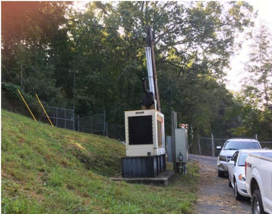
Replace generator in existing location
