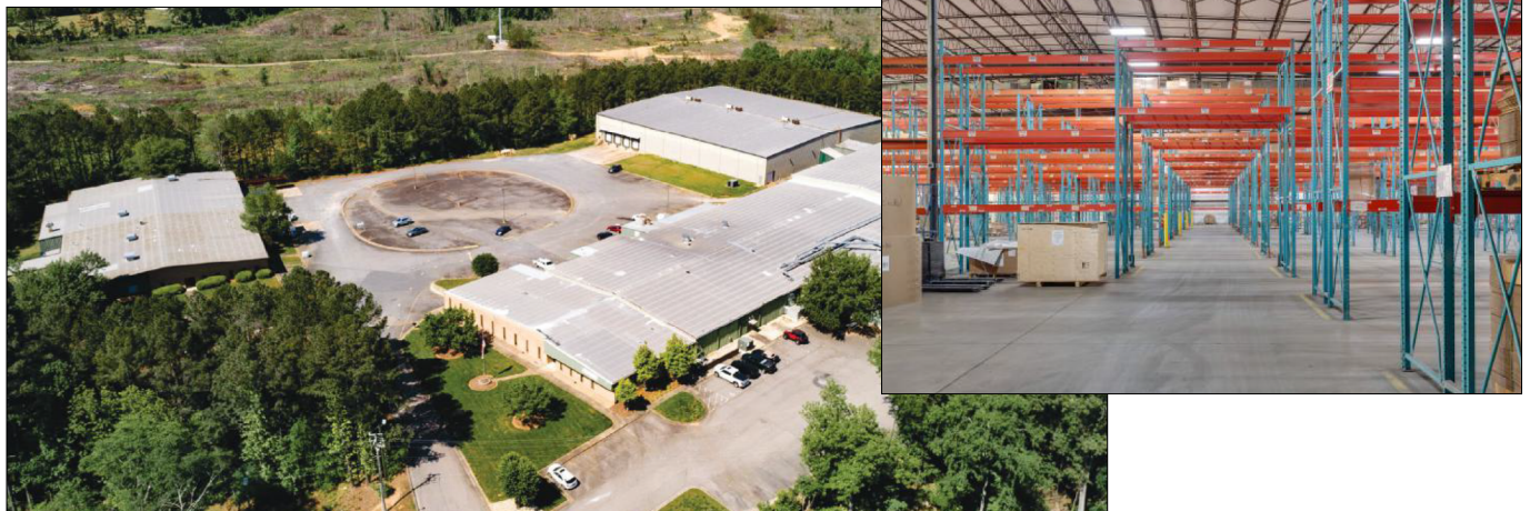
Former Paperworks Facility, Mt. Gilead, NC
