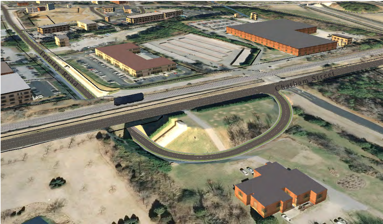
Railroad bridge over Trinity Road at new crossing location with loop ramp to Chatham Street
