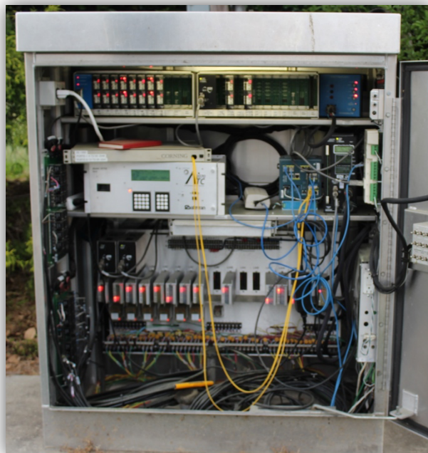
Figure 2.1: 2070 controller with MMU in NEMA TS 2 cabinet
