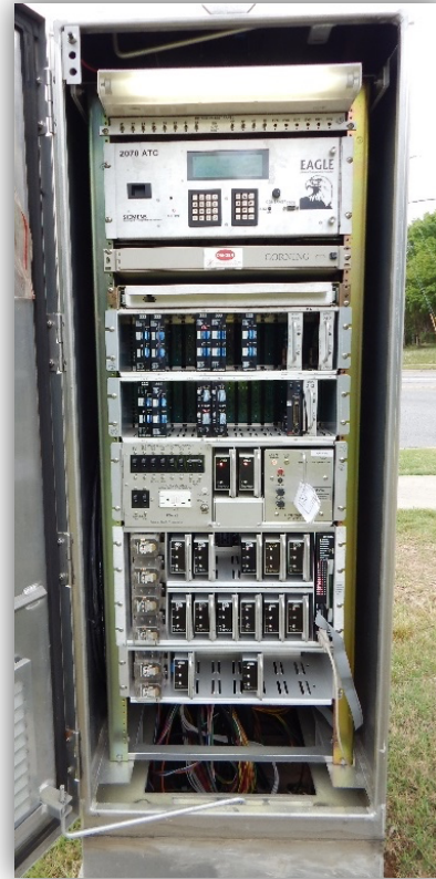
Figure 2.2: 2070 controller with CMU in 332 cabinet
