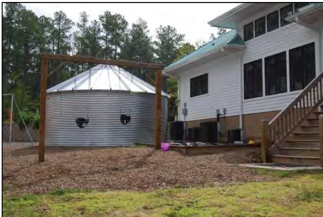
Examples of innovative stormwater management practices (from top to bottom): pervious pavement, parking lot draining to a bioretention cell, and cistern used for rainwater harvesting (Sources: NCSU (2009) and Tetra Tech)
