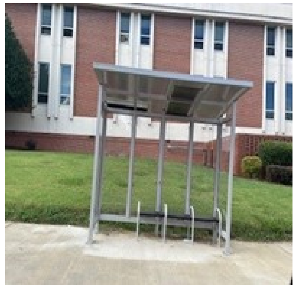
Newly Installed bus shelter in partnership with GO Durham along Lawson Street next to NCCU Campus.
