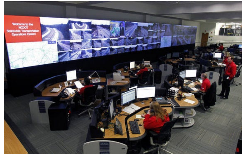
North Carolina's State Traffic Operations Center
