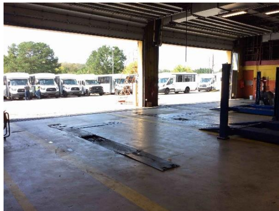
Decommissioned in-ground lifts have not been removed and filled
