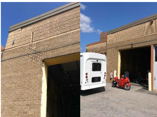
A portion of the facility is separating from the main structure. The site is located on an old land fill which is unstable
