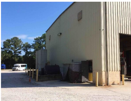
Oil, gasoline, and diesel are stored outside the facility. Fuel is only plumbed into the building; buses are filled off-site.
