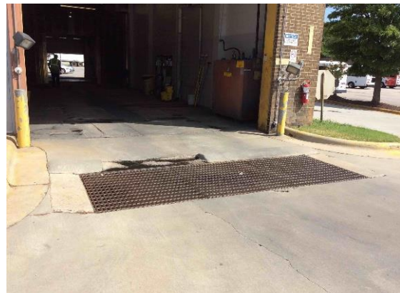
Numerous areas on the site have begun to sink due to the unstable subgrade, such as outside of the old wash bay
