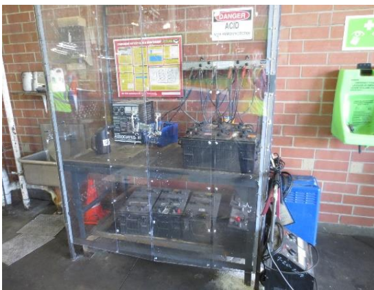
Batteries are currently stored in a locked cabinet instead of in a dedicated storage/charging room
