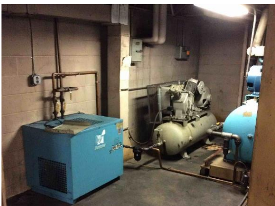
Two compressors are used to supply the maintenance shop; compressors are located on the mezzanine
