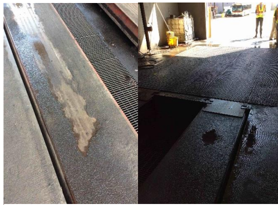
Traction coating on the lift in the Chassis Wash needs recoating
