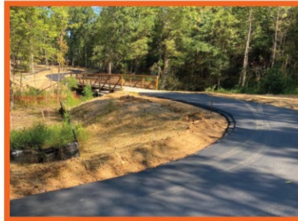
Utley Creek Bridge Crossing
