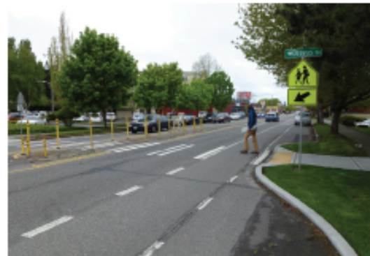
MEDIAN REFUGE ISLAND
