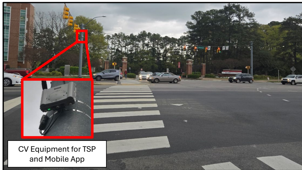
Western Blvd. and Avent Ferry Rd. Traffic Signal and CV Equipment for TSP Operations and Mobile Application for Pedestrians / Motorists
