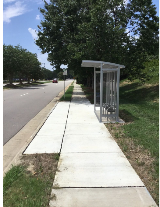
GoTriangle bus stop at McCrimmon Parkway and Airport Boulevard. This stop received a shelter, seating, and an ADA accessible landing area to the curb in 2021.
