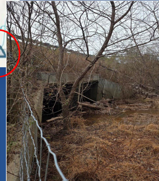
Little Branch Creek NC 540 NB
