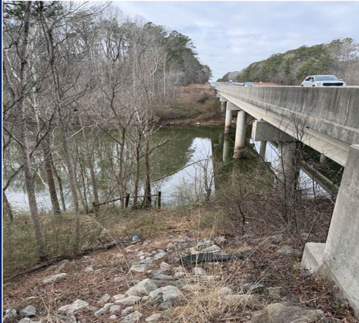
Haw River Bridges over US 1 Condition: Fair Opportunity: improvements during future maintenance
