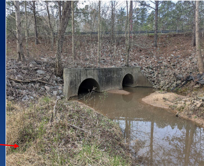
Davis Drive Culvert (Not Formally Assessed)
