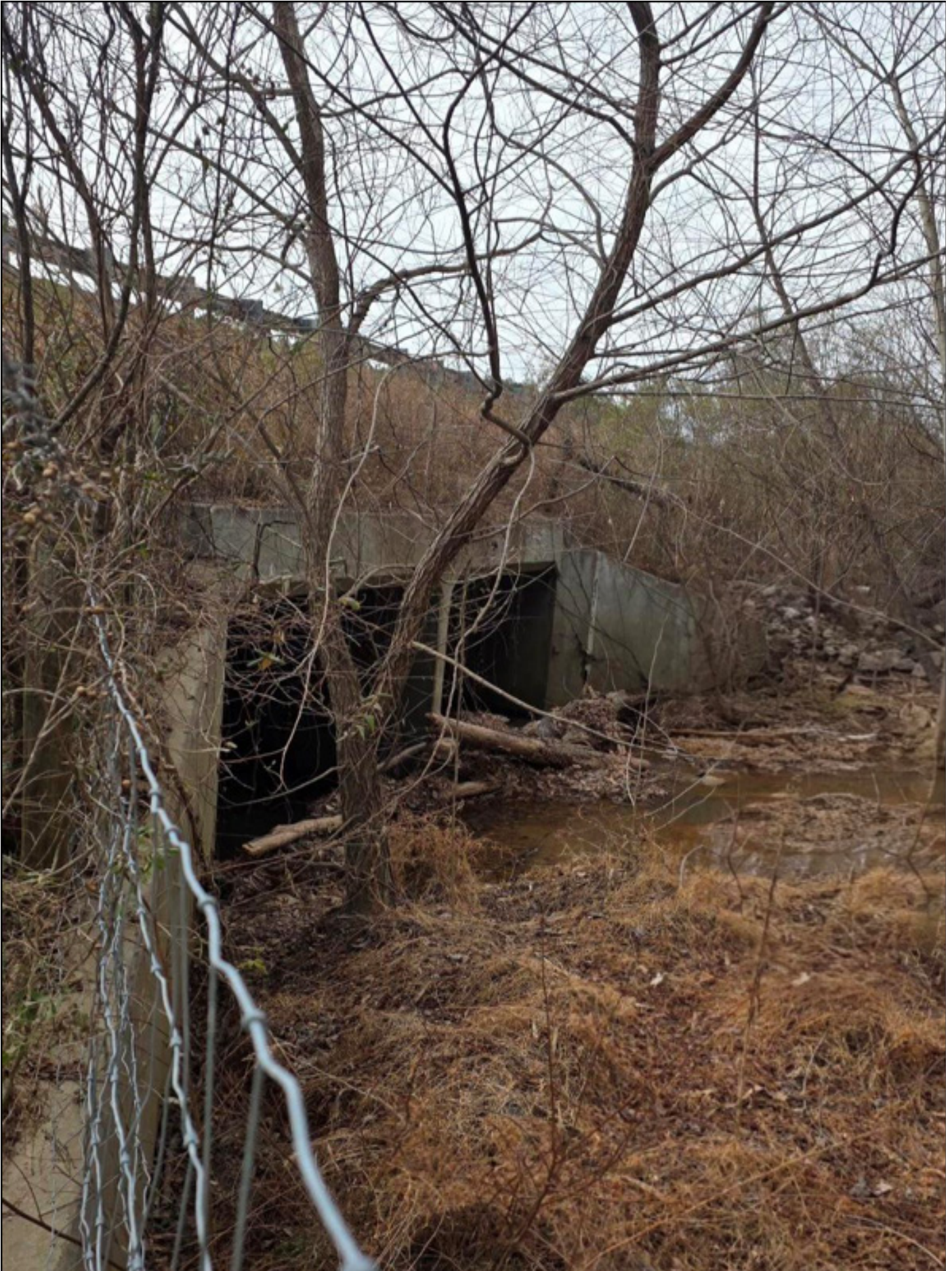
Figure 8: Little Branch Creek Culvert
