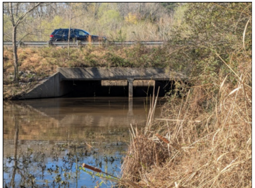
Figure 16: Davis Drive Culvert
