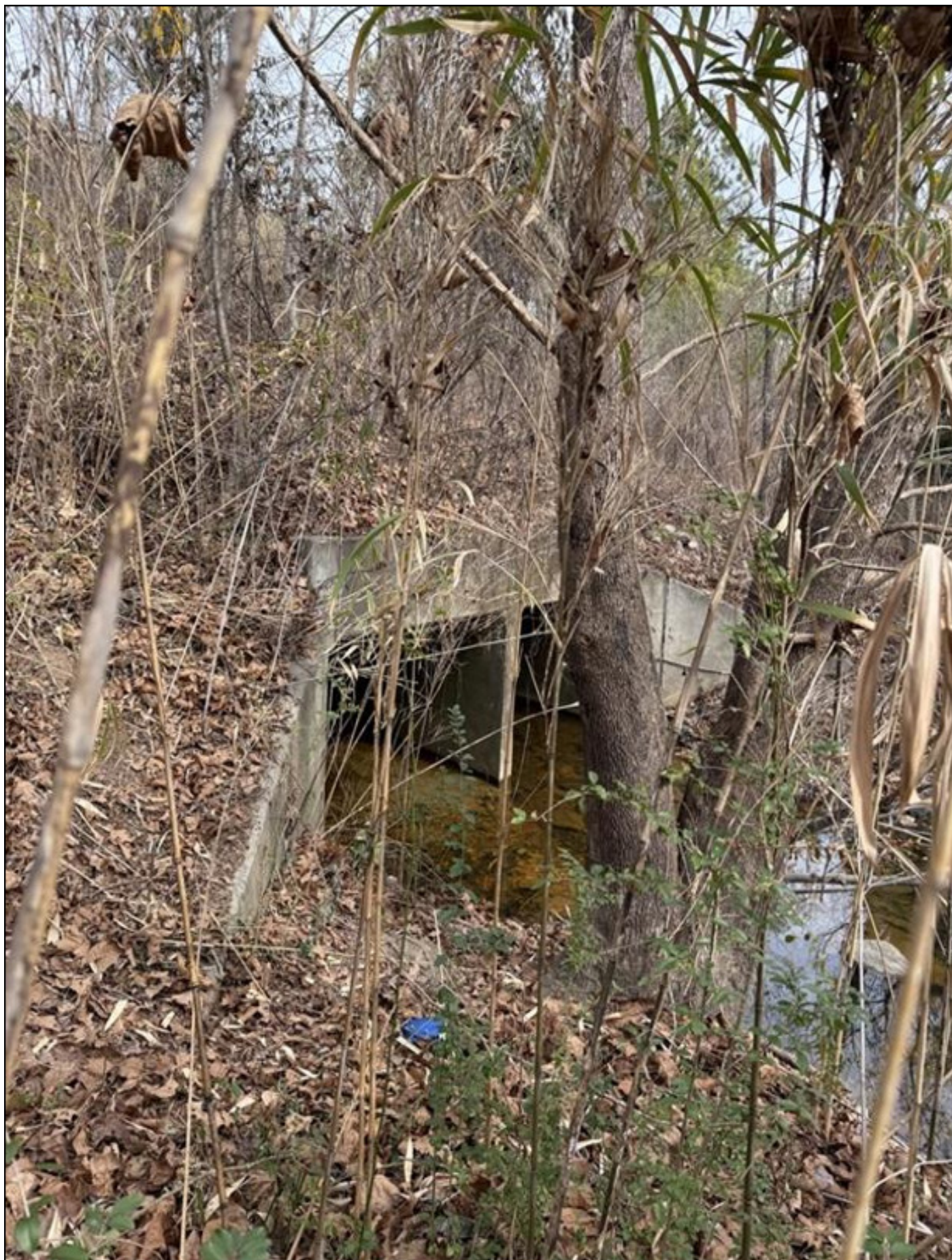
Figure 10: Big Branch Creek Culvert
