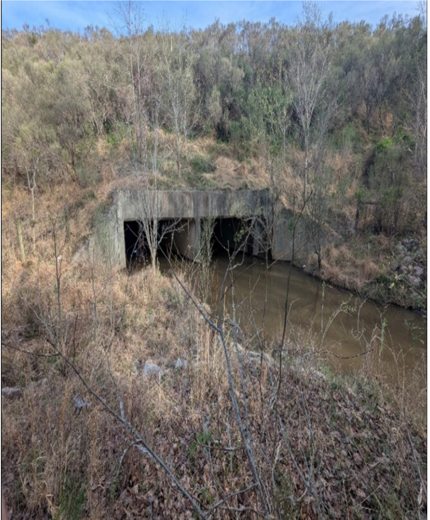
Figure 14: N.C. 540 Northbound Ramp
