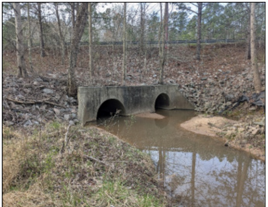
Figure 17: Davis Drive Culvert (Not Formally Assessed)
