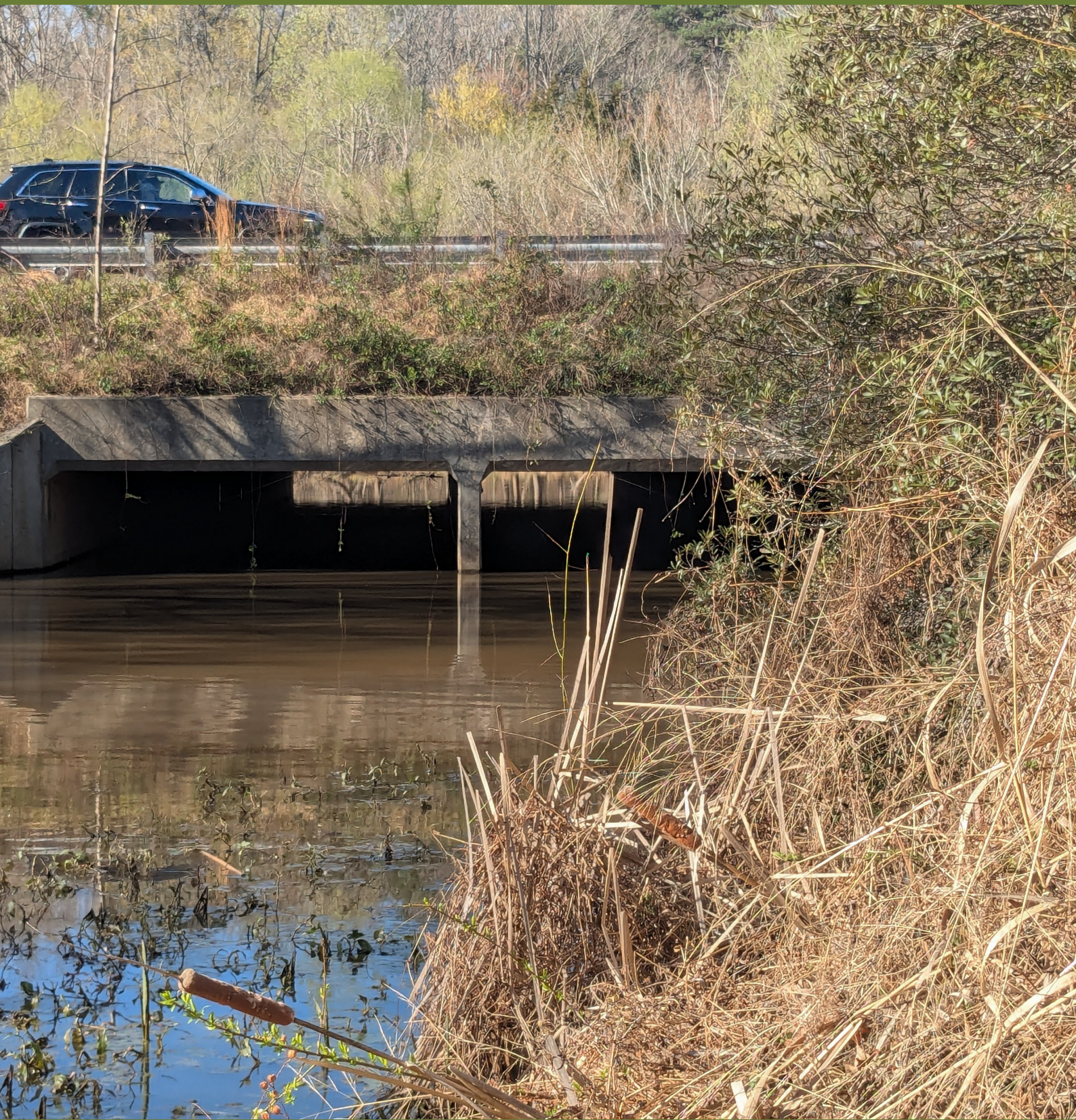
Culvert at Davis Drive (2026)
