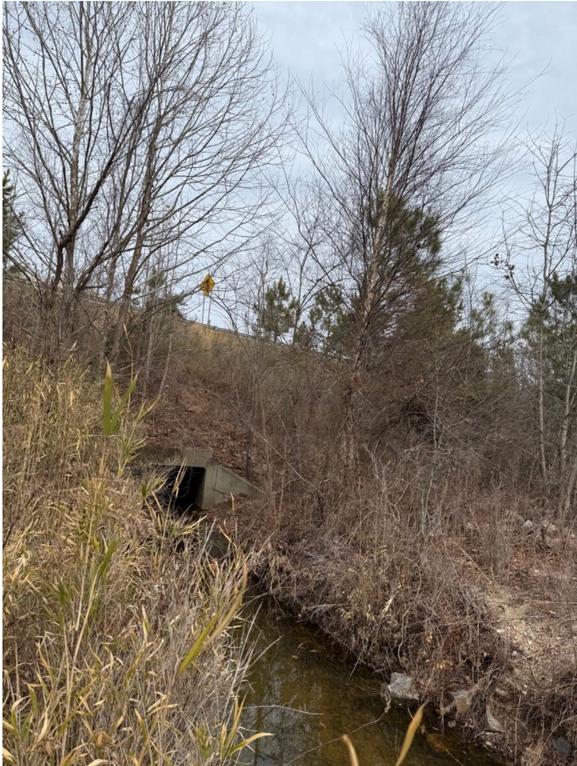
Culvert at Big Branch Creek (2026)
