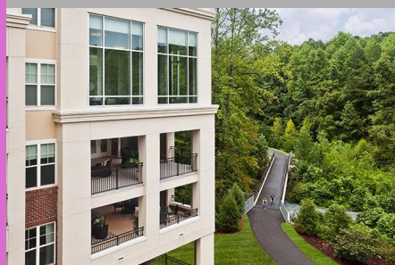
Trail Oriented Development
