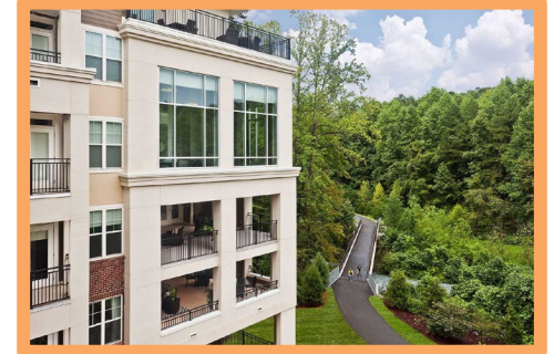
Trail Oriented Development
