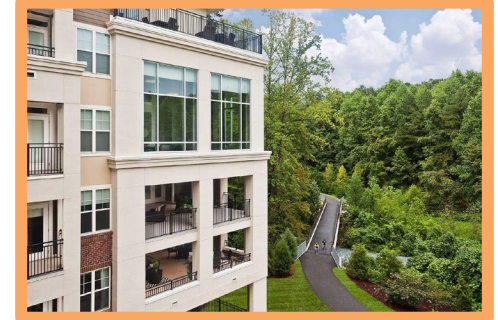
Trail Oriented Development
