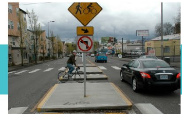
Median Refuge Island
