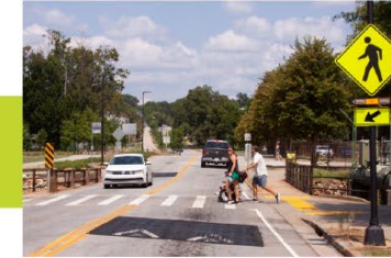
Rectangular Rapid Flashing Beacon (RRFB)
