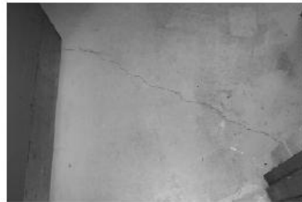
Concrete floor needs painting
