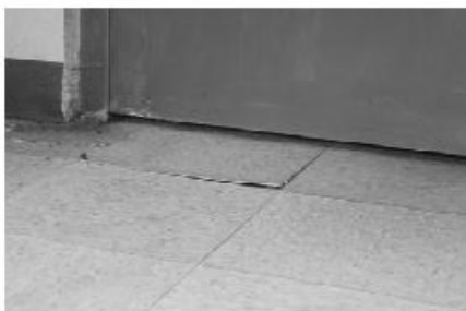
Tile and Door – Inmate Property Room
