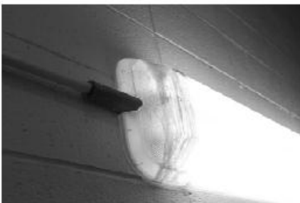
Chalky substance for roof leak
