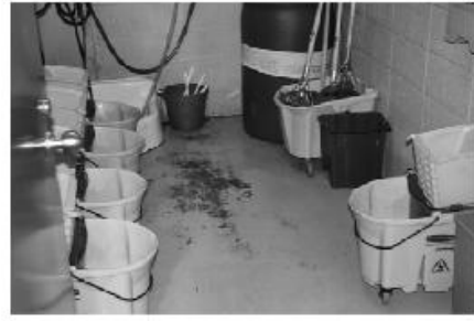
Maintenance Issues – Floor painting
