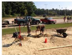
Digging holes for court net posts, mixing and pouring concrete
