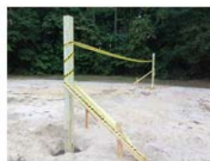
Posts set, leveled and secured
