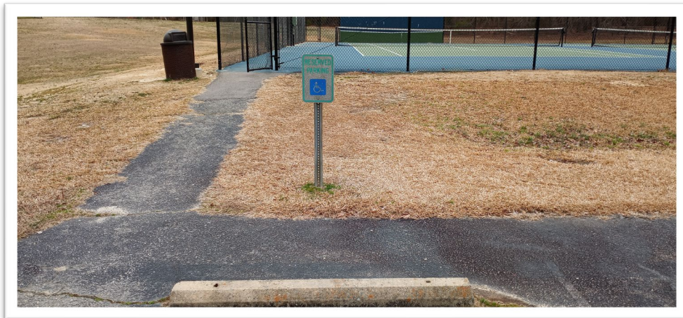
Figure 19: Tennis Court Accessible Parking Signage and Access Ramp
