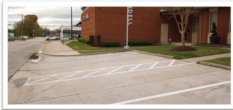
Figure 6: Town Hall Parking, Sideview
