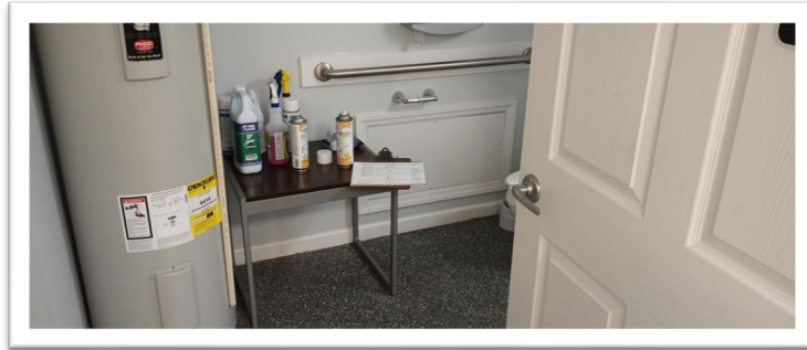
Figure 81: Public Works Single User Toilet Room
