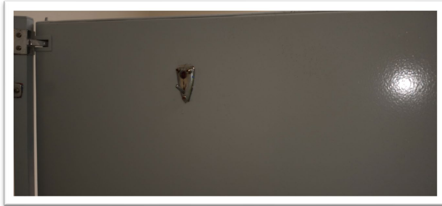
Figure 60: Senior Center Women's Main Bathroom Coat Hook
