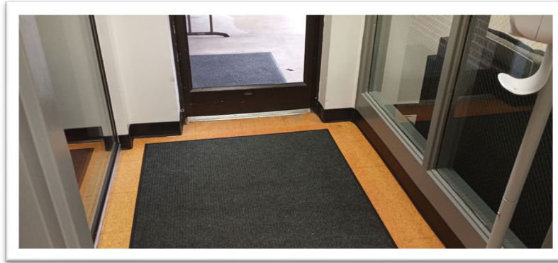
Figure 53: Senior Center Front Door Mat
