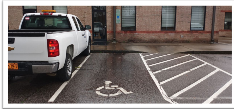
Figure 32: Community Center Accessible Parking, Access Aisle, and Curb Ramp
