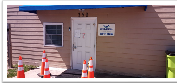
Figure 79: Public Works Accessible Entrance
