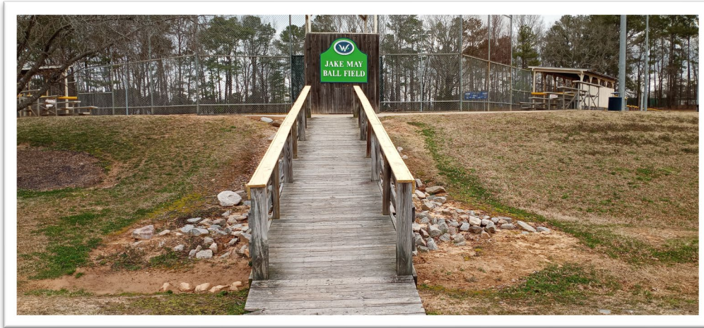
Figure 20: Jake May Ball Field Access Ramp
