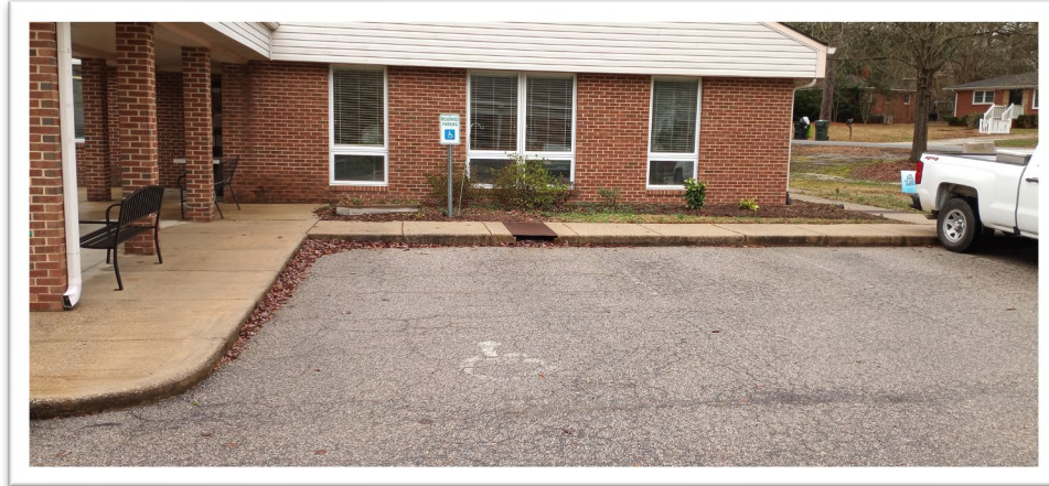
Figure 48: East Wake Senior Center Accessible Parking Space
