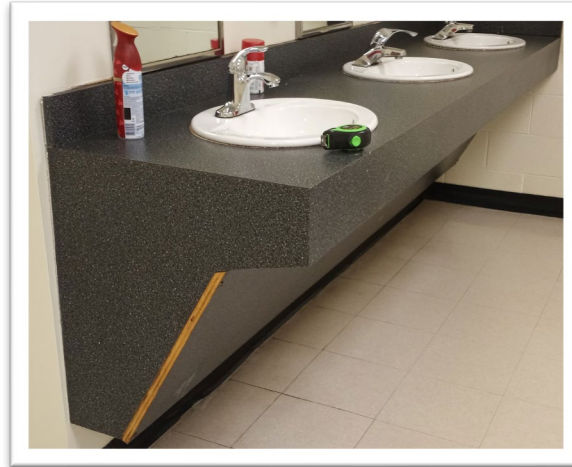
Figure 40: Bathroom Sink Accessibility View
