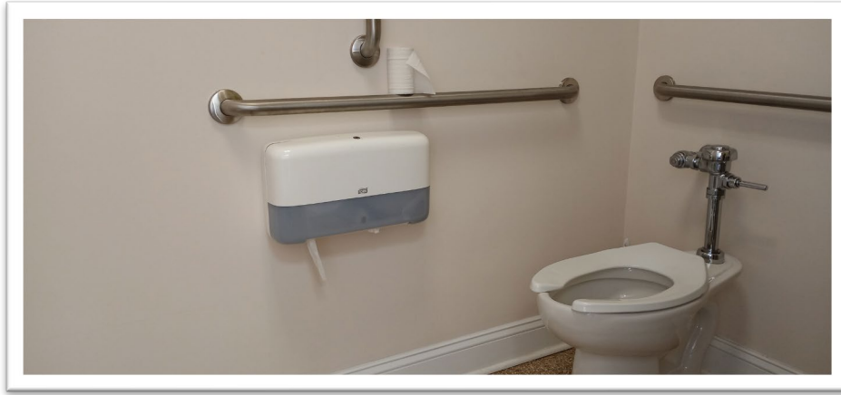
Figure 15: Accessible Bathroom Toilet Paper Dispenser
