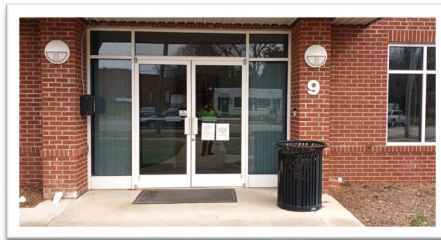
Figure 73: Police Department Accessible Entrance
