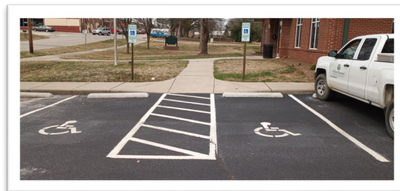
Figure 71: Police Department Accessible Parking Spaces
