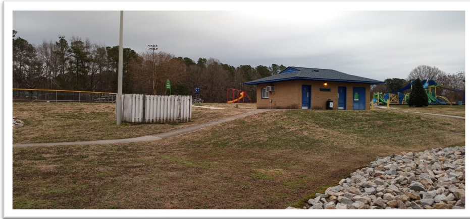
Figure 22: Concession Stand Access Ramp
