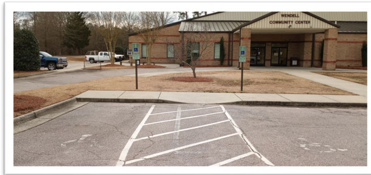
Figure 33: Community Center Front Entrance Accessible Parking, Access Aisle, and Curb Ramp
