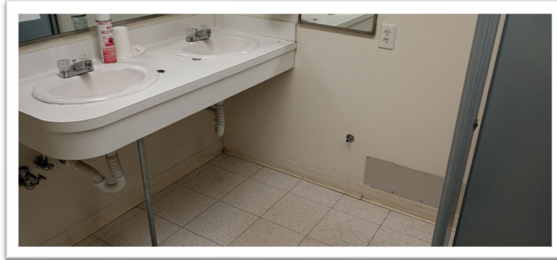
Figure 58: Senior Center Men's Lobby Bathroom Clearance
