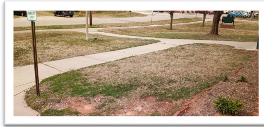
Figure 72: Police Department Accessible Path
