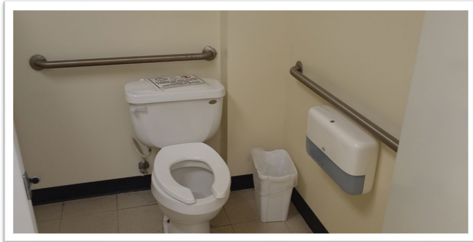
Figure 44: Main Lobby Women's Bathroom Accessible Stall
