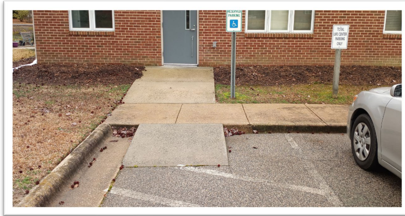
Figure 51: East Wake Senior Center Side Access Ramp
