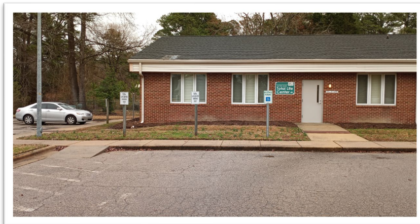
Figure 50: East Wake Senior Center Front Corner Ramp
