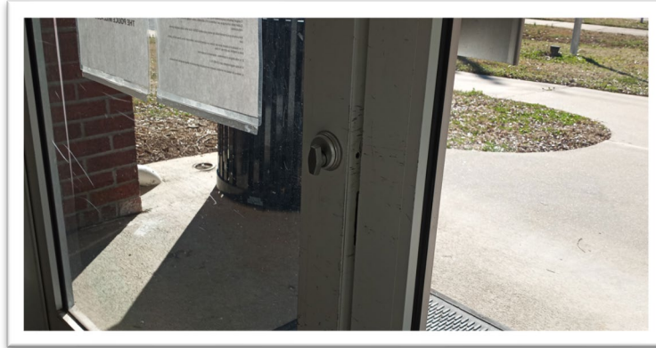
Figure 75: Police Department Accessible Entrance Door Lock
